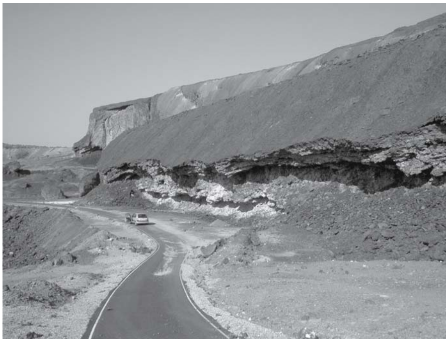
Fig. 2.8. Face of the Río Tinto smelting slag dump, Spain. Mineral efflorescences commonly occur as white sulfate salt precipitates (gypsum, epsomite, hexahydrite, bloedite, copiapite, roemerite) in protected overhangs and at seepage points at the base of the slag dump. The slags generate ephemeral drainage, which runs from the dump into the Río Tinto and contributes to its acidification and metal load
