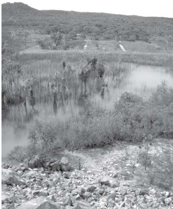
Fig. 3.14. Wetland at the Horn Island gold mine, Australia. The wetland has failed because an adjacent damwall was constructed using acid generating waste rocks (foreground), which resulted in significant AMD and caused plant death
