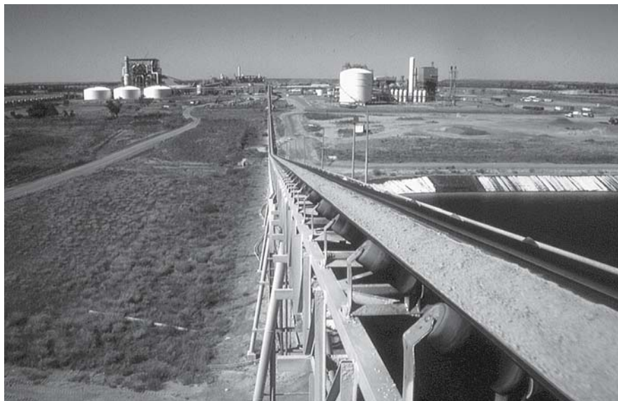
Fig. 7.4. View of parts of the fertilizer production facility at Phosphate Hill, Australia. Ammonia plant ( far right ), phosphoric acid facility ( centre ), granulation plant ( left ), and rail loadout facility ( far left ). A conveyer belt delivers phosphogypsum to the stack
